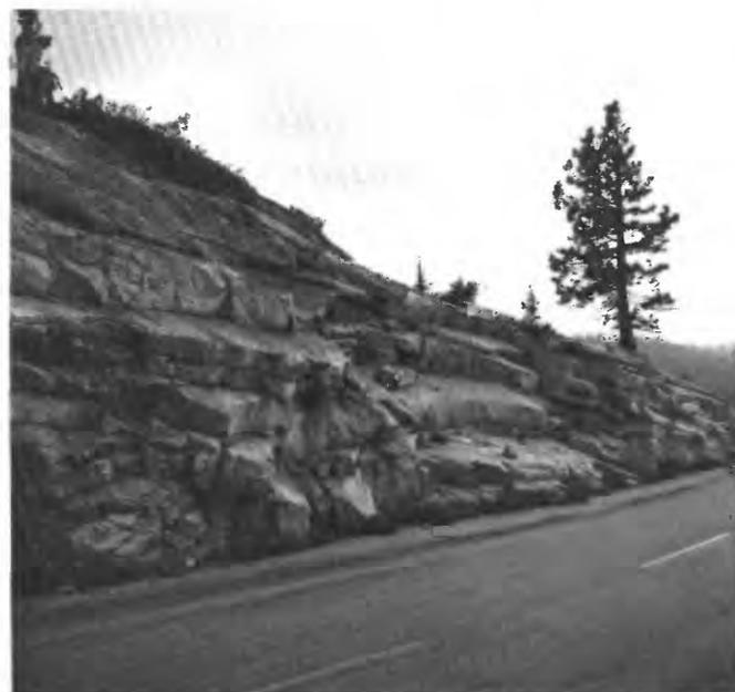
FIGURE 25.—Sheeting in the Sentinel Granodiorite due to unloading by erosion. Roadcut along California Highway 120 (Tioga Pass Road).
